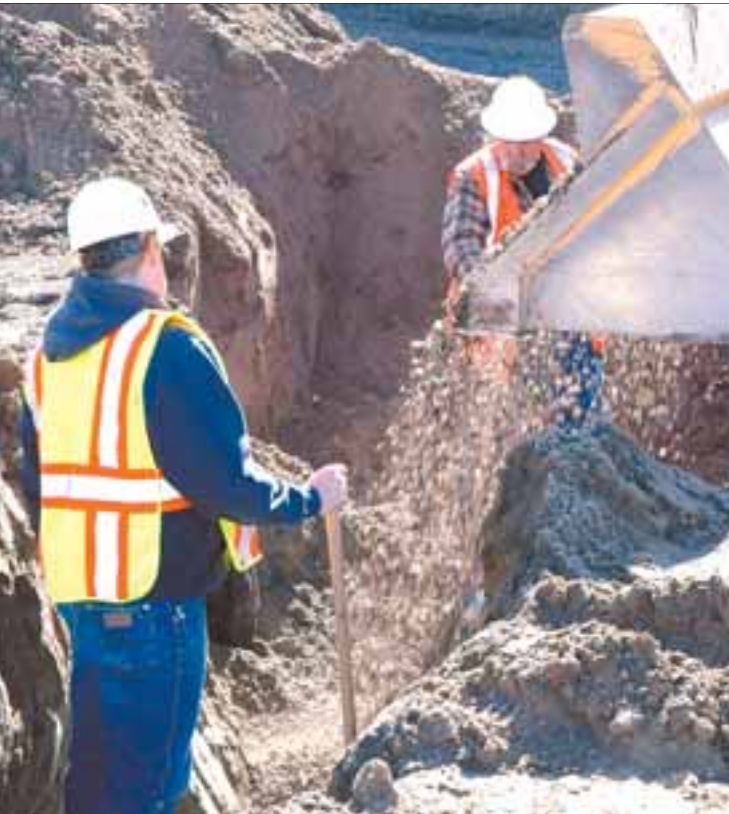
Uria Pump employee Terry DeWeese, right, shovels gravel from a bucket Thursday as he and co-worker Mike Riley fill in a trench after setting six-inch sewer pipe for Dairyland Seed Co.
